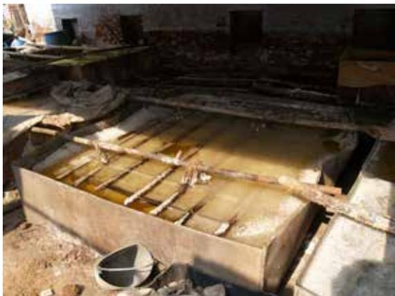
**Figure 5. The settling tank with bamboo lattice on top**
