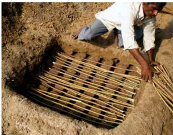
**Figure10. Laying a layer of sticks over the bricks**
