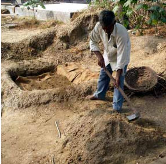
**Figure 12.** The saltpetre soil is put over the sacking
